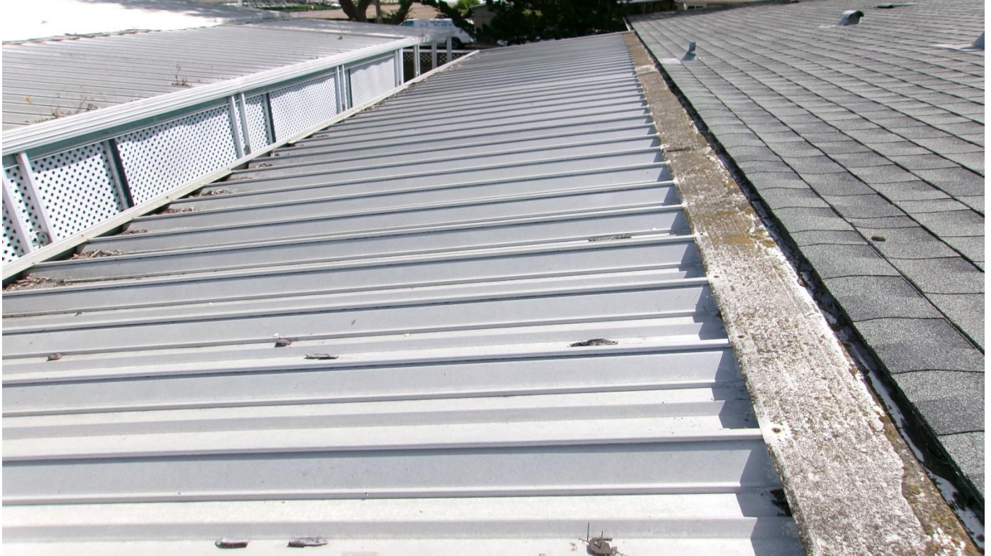
View of the carport cover surface.
