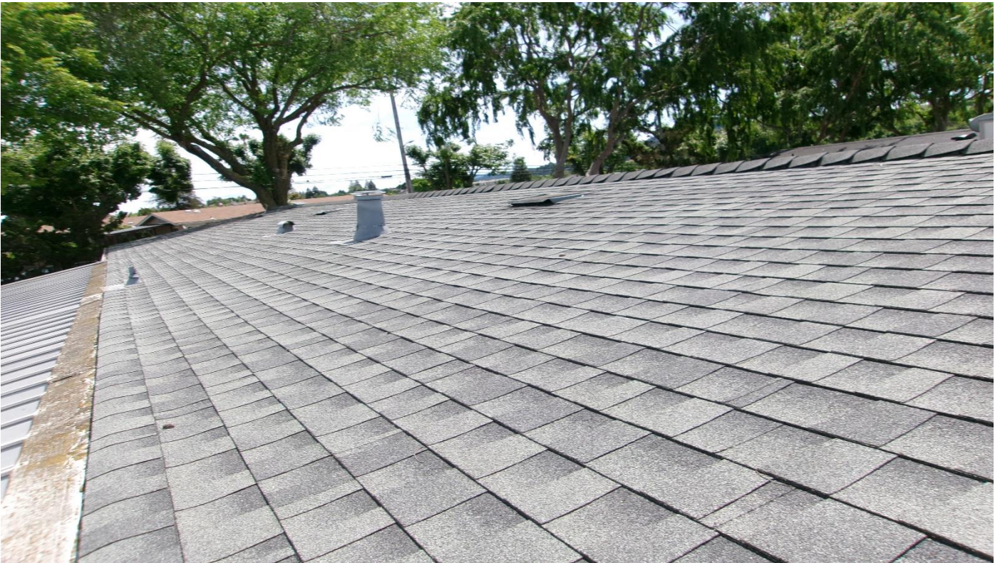
View of the roof surface.
