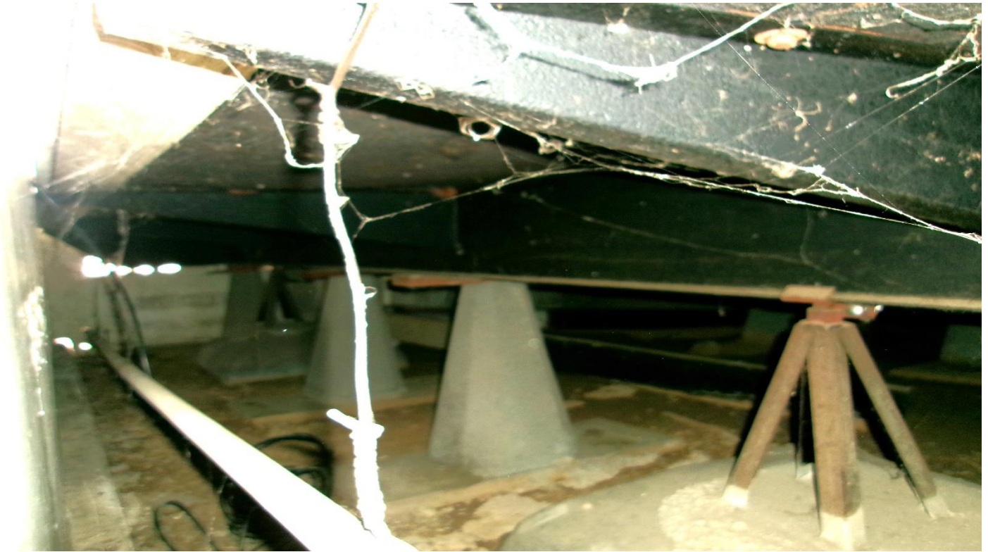
View of foundation support at the sub-area.
